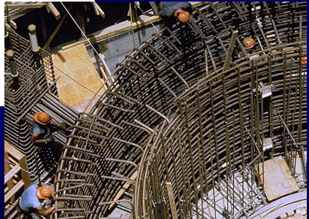
Containment Building Wall Construction
