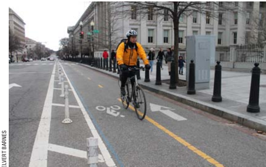
An example of the successful and well-used bike lane infrastructure along 15th Street, a major downtown corridor in Washington, D.C.
