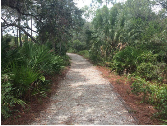
Trail section made of compacted limestone shell
