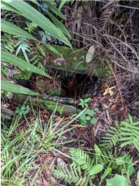
Culverts observed within the property
