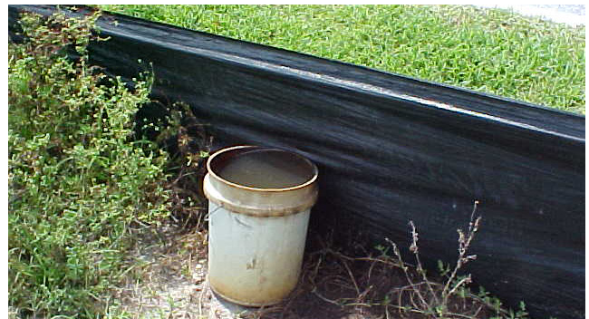
Avoid Leaving Hazardous Materials Unsecured
