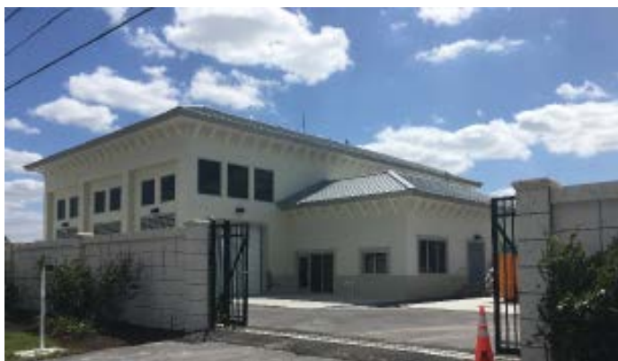
Master Pump Station 306 3935 Thomasson Lane Drive
