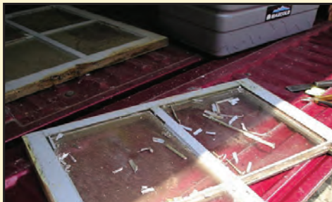
Window frames broken
