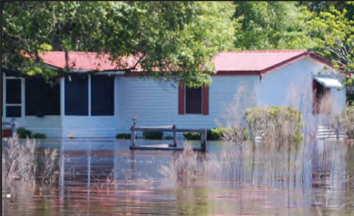
Minor: 10," standing water, Single Family (SF)
