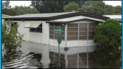
Major: 3," standing water, Manufactured Home (MH)
