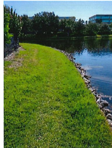
Figure 2: Rip-rap has been installed around approximately half of the existing lake bank on Lake 1-3.
