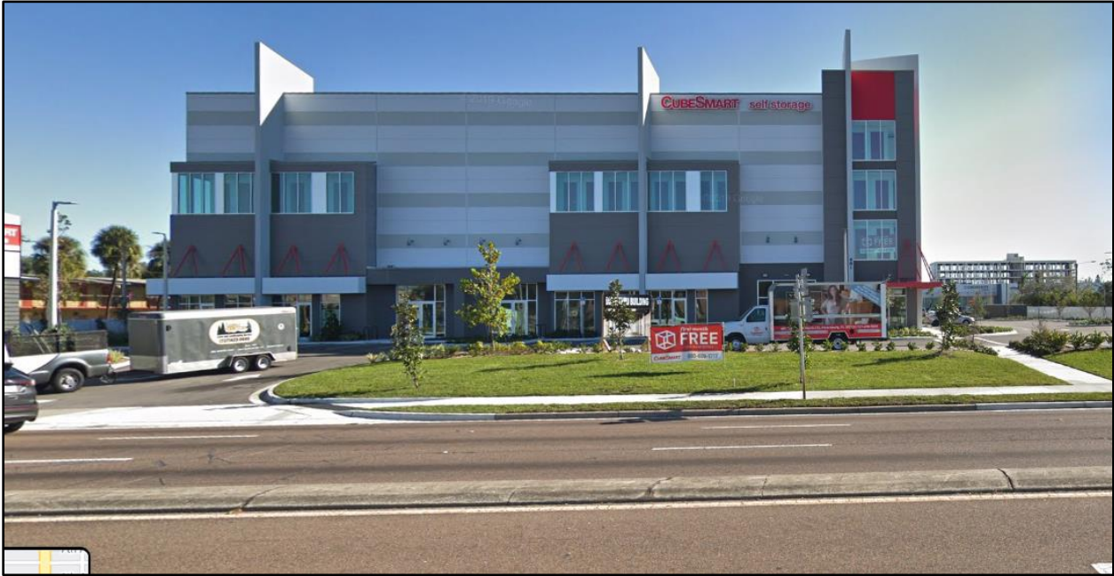
401 34 th Street North in St. Petersburg, FL
