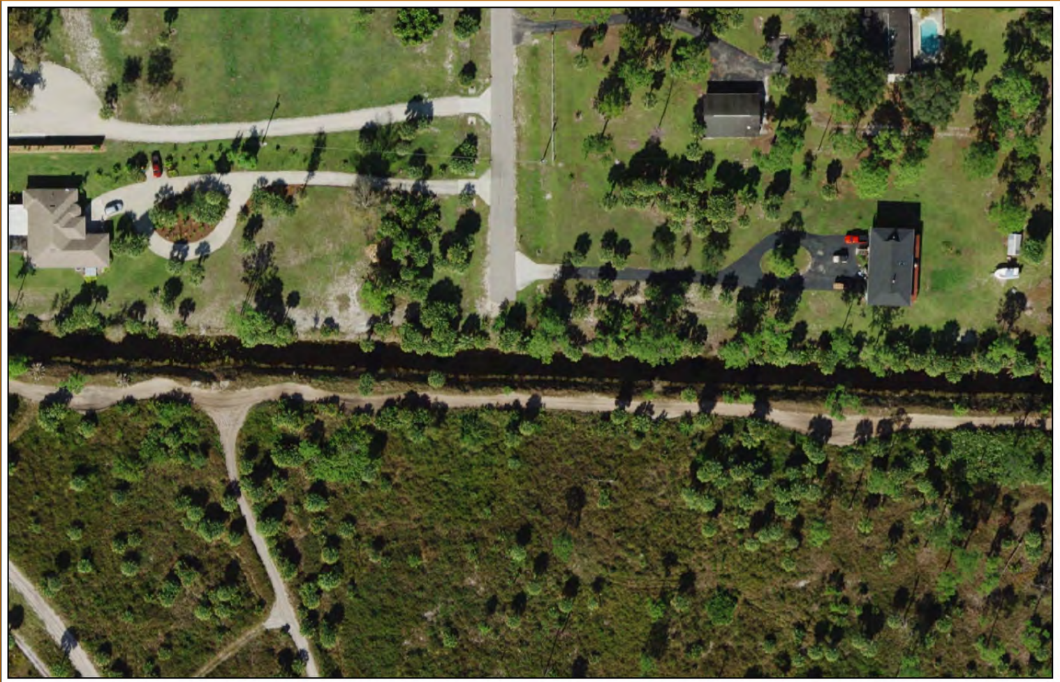
Location of Bridge #9: Existing Condition
