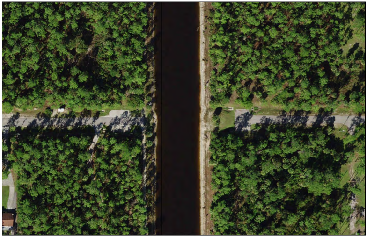
Location of Bridge #11: Existing Condition
