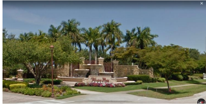
Example of monument sign and gateway feature with landscaping from Treviso Bay community. Image Source: Google Maps
