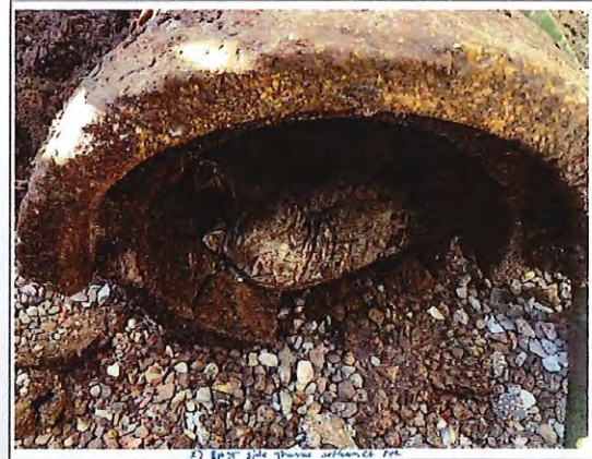
Damaged 24' stormwater pipe
