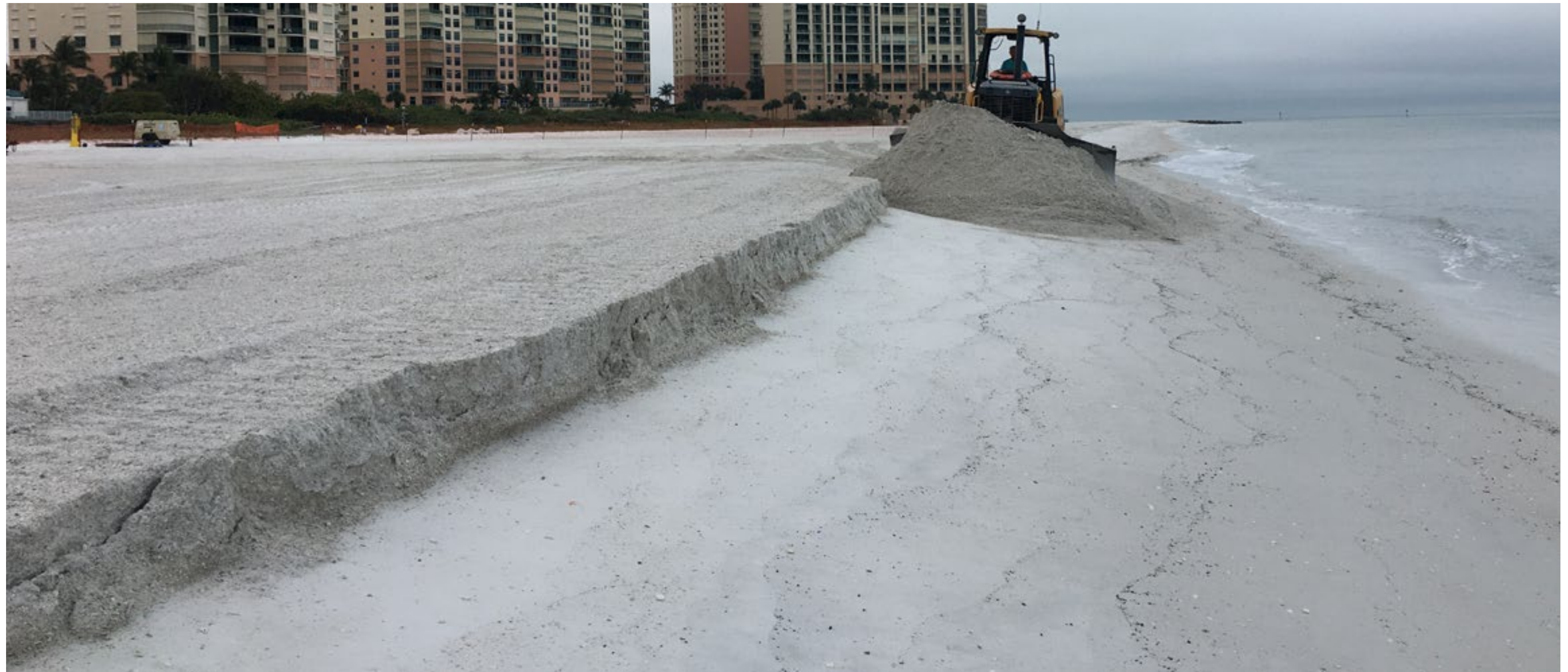
Beach Dredging and Renourishment Project at Caxambas Pass, Marco Island
