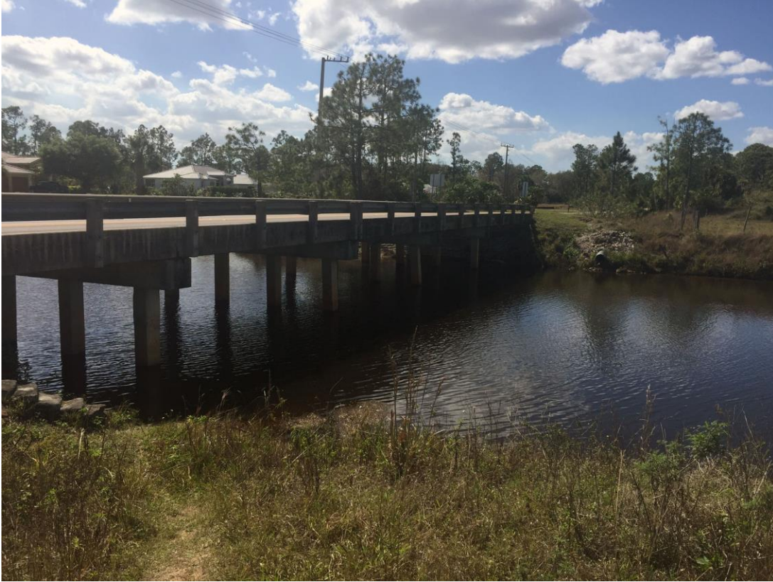
Figure 15. Easternmost bridge on Oil Well Road, looking northeast.
