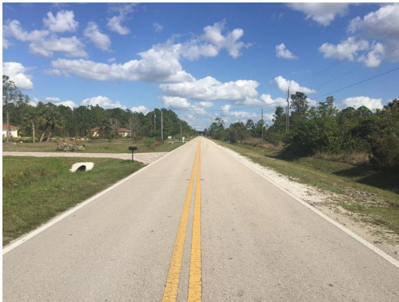
Figure 7. Randall Blvd, looking east in project corridor.
