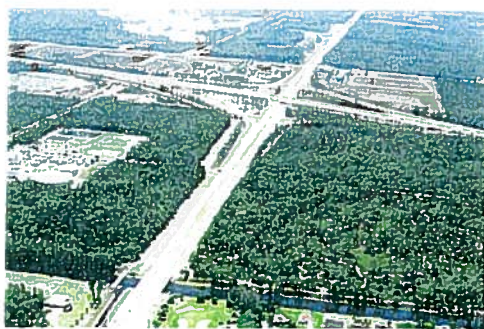
Looking southeast across Activity Center #9.
