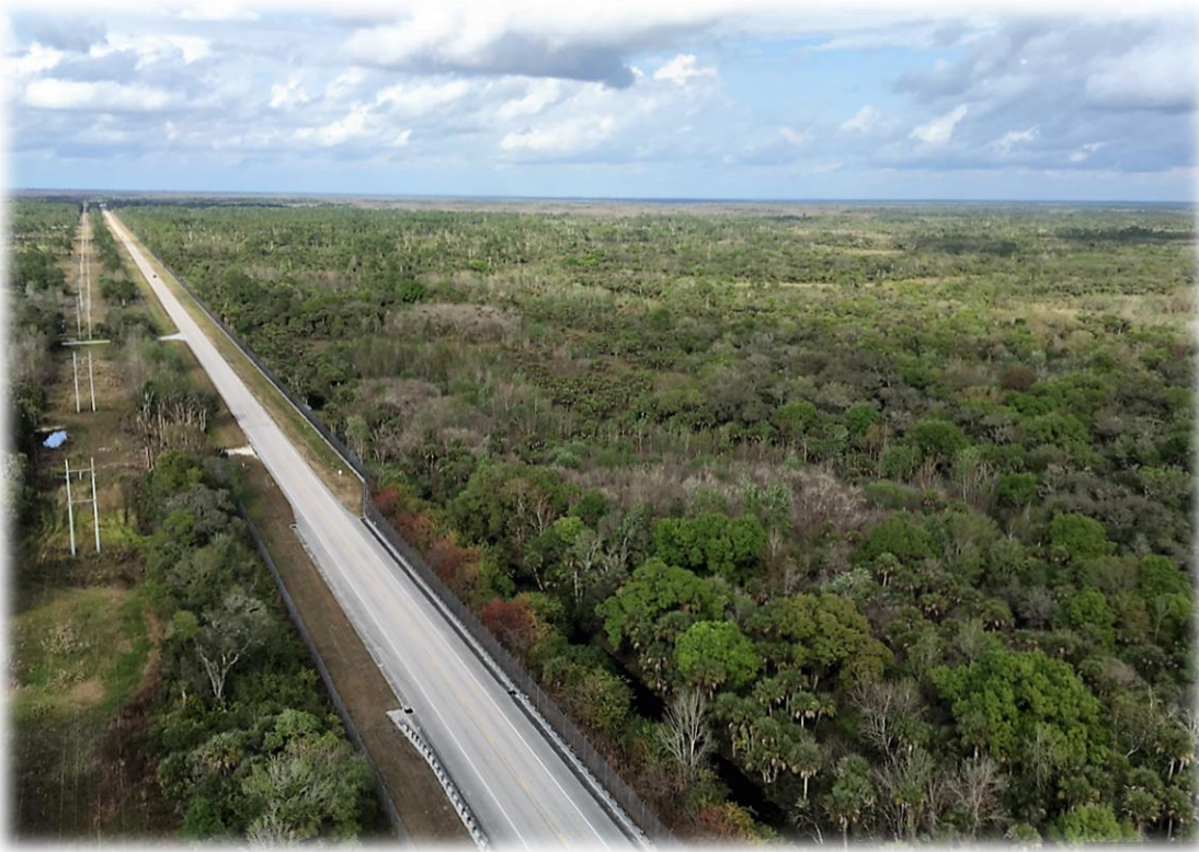
Figure 2: Aerial view of SR29 road and canal corridor about 1 mile north of I-75, looking north
