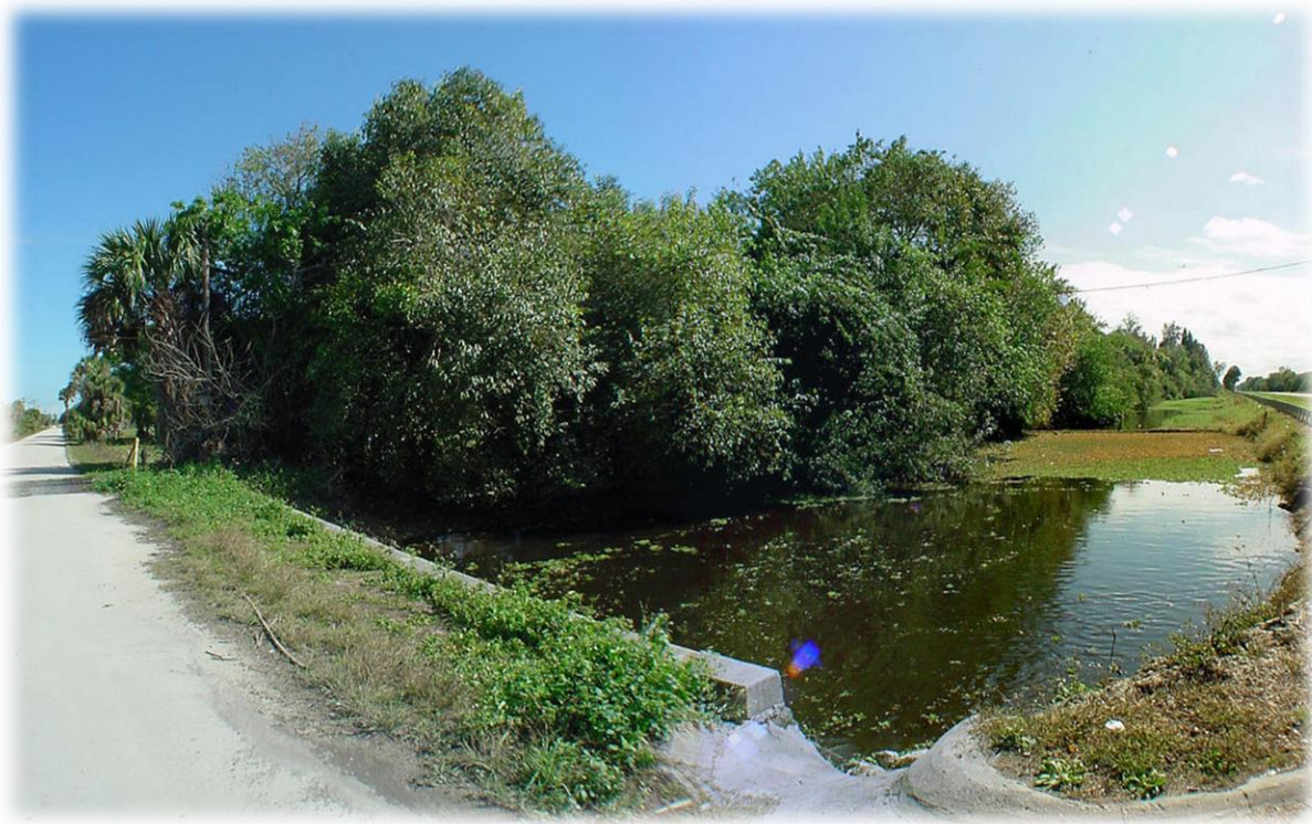
Figure 11: SR29 Canal looking south from Sunniland. The canal will remain a drainage, water quality and environmental problem, and will worsen in the future without action.
