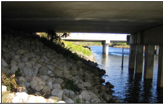
Wildlife Crossing Improvements – Miller Canal and I-75
