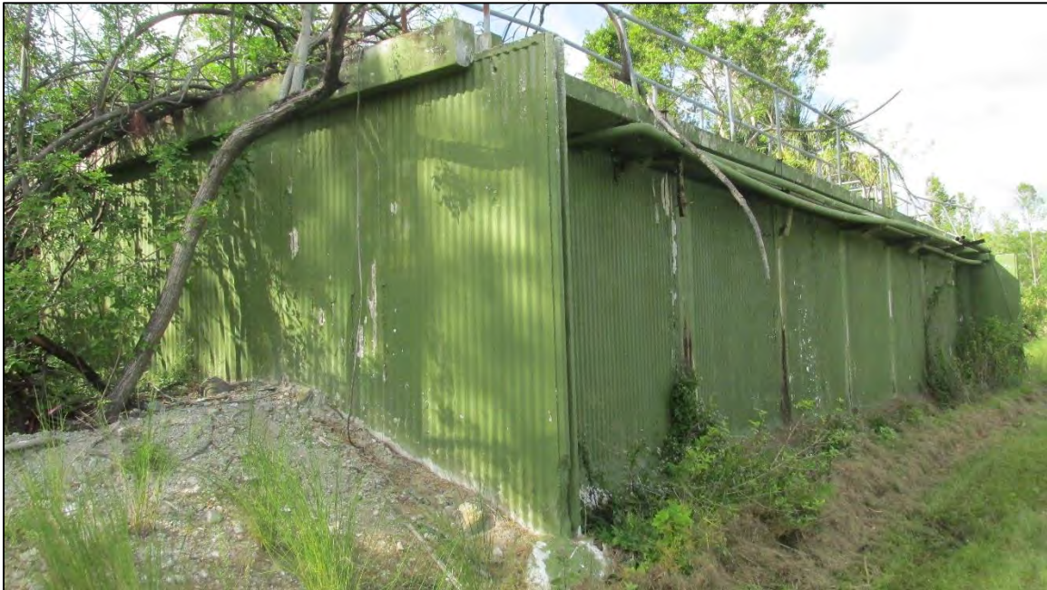
Photo 2. Old water treatment facility – to be removed
