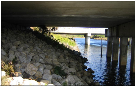
Wildlife Crossing Improvements – Miller Canal and I-75
