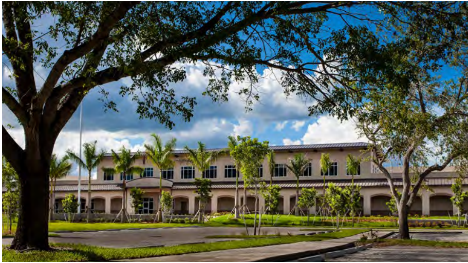
LeeSar Regional Service Center completed by SchenkelShultz & GATES Construction
