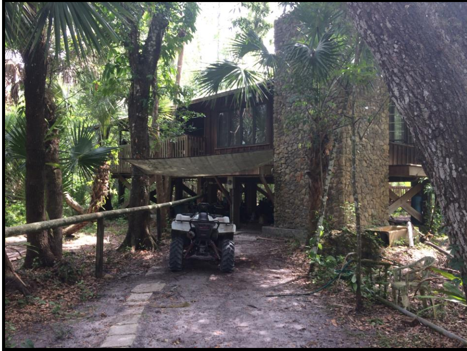
Photo 4: Gore home site structure. Photo taken May 30, 2017.
