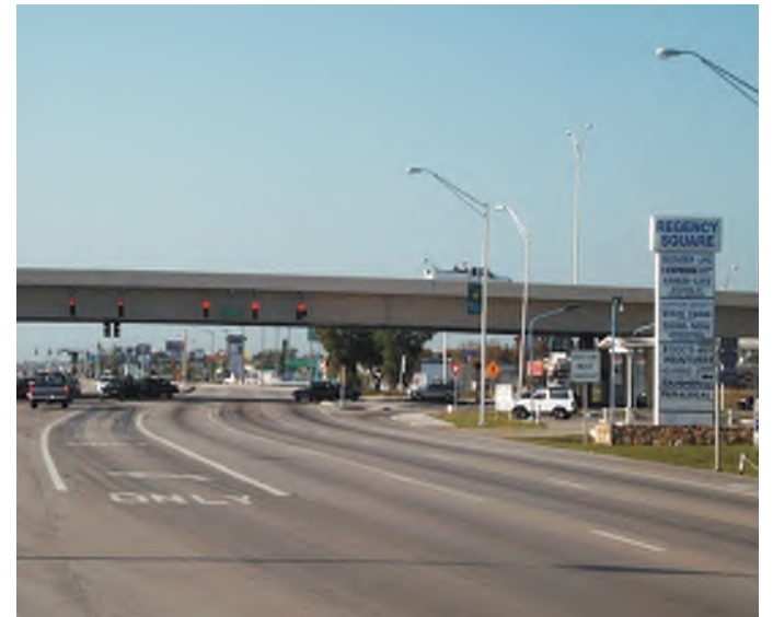
Grade-separated interchange in Lee County
