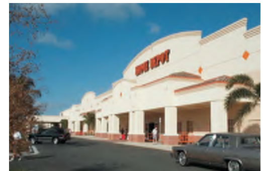
The built result
