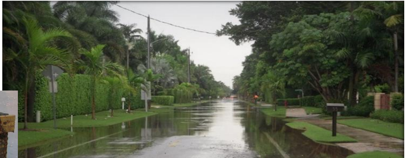
Flooding of Gulf Shore Road (Near 2 nd Ave N/Outfall 8, Sept 2015)
