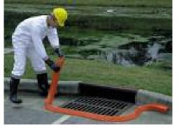
1. **Containment Booms** – Protective barriers can be placed around a storm drain in order to prevent water from entering the drain. They are normally used in order to prevent wastewater from entering a stormwater drain and to pool the wastewater around drain for later collection. However, one potential problem with berms is that they can be ineffective or less effective when the storm drain is located at the bottom of a slope or if there is a large amount of wastewater generated.
