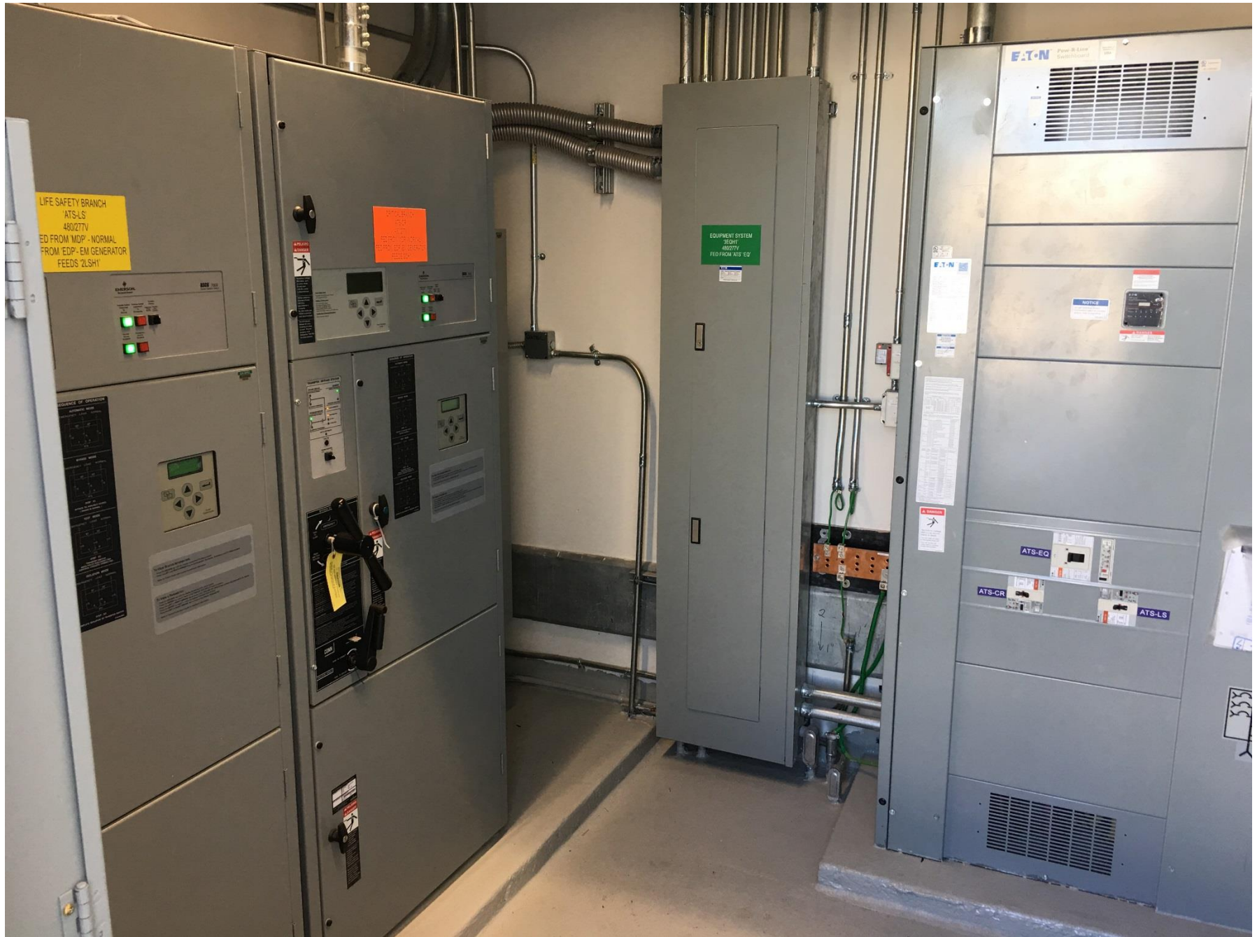
502- Final electrical work performed.
