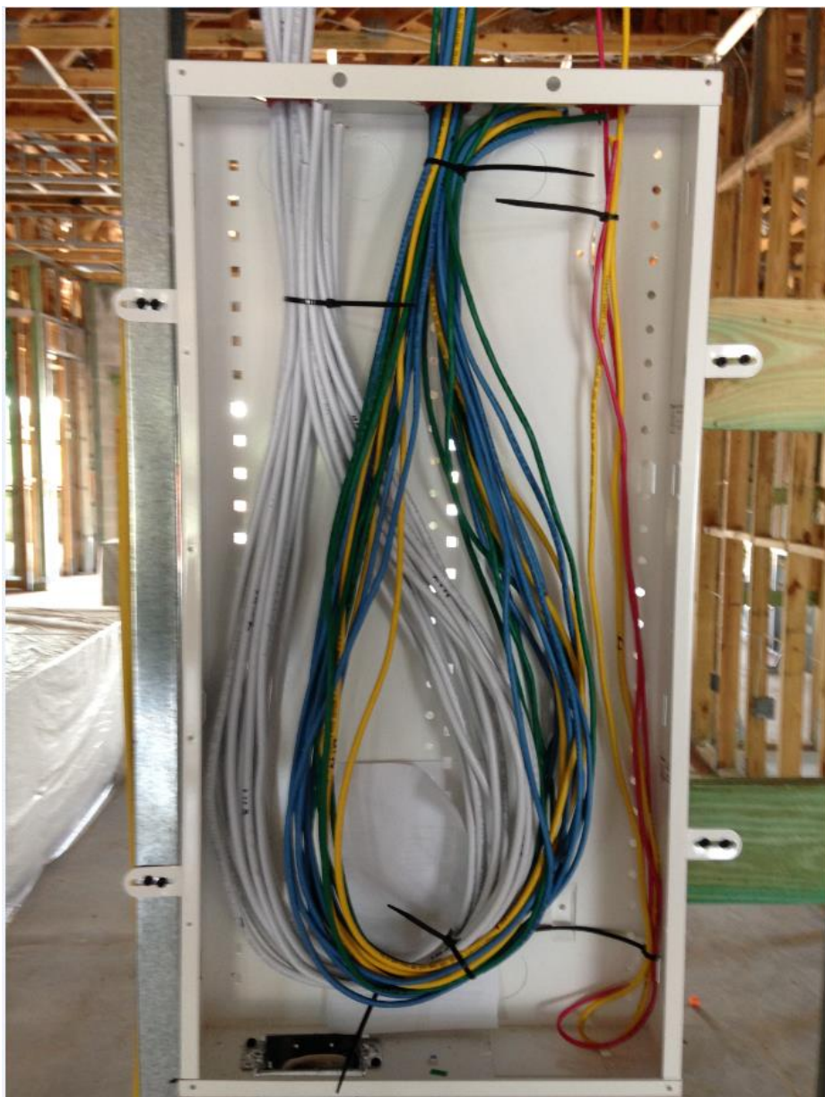
510- Primary alarm system work performed, before insulation and drywall is installed
