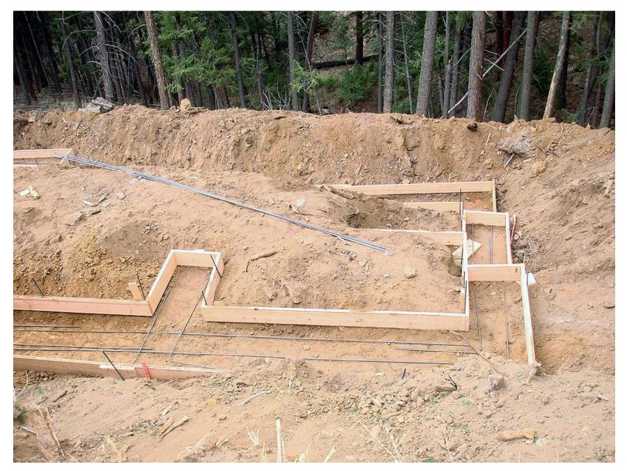
**DESCRIPTION:** When regular continuous footings are used, call for inspection when footings are excavated, neat, clean, dry and forms are in place, level, braced and reinforcing bar if required is in place and tied. Reinforcing bar must be suspended in place a minimum of (3) inches above the soil. If footings are on fill, you must have a compaction report by an engineer on job site at time of inspection.
