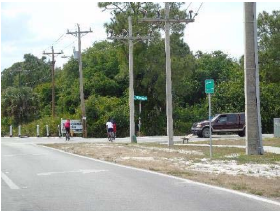
Bus shelters (shown below) will be provided at CAT transit locations.
