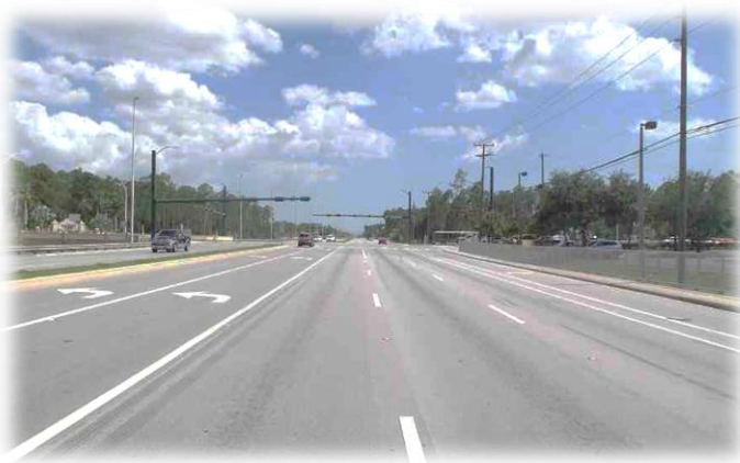
Completed Collier Blvd II Segment
