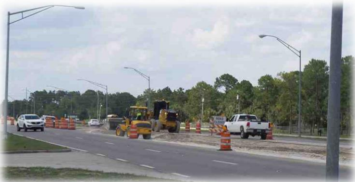
Construction on Collier III - Phase I
