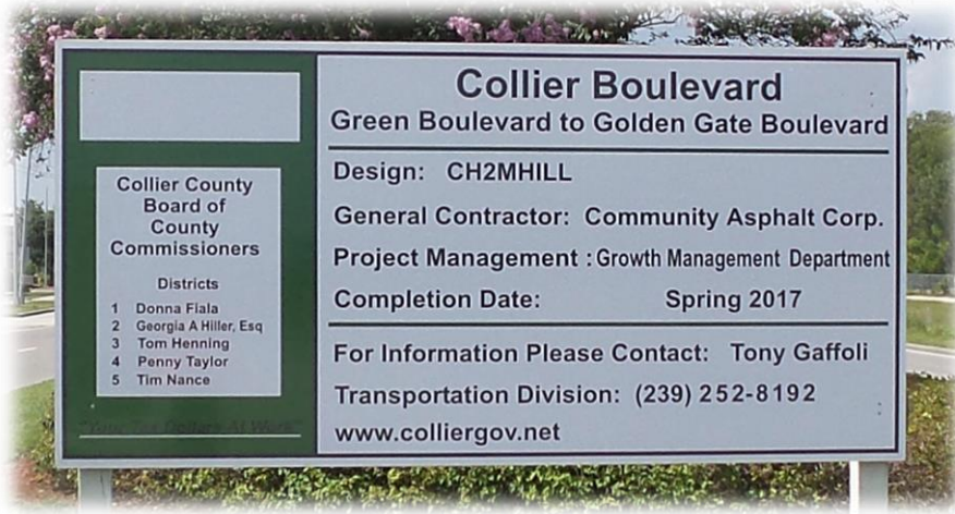
Collier Boulevard Project adjacent to TIGER project, under construction (Collier III, Phase I)
