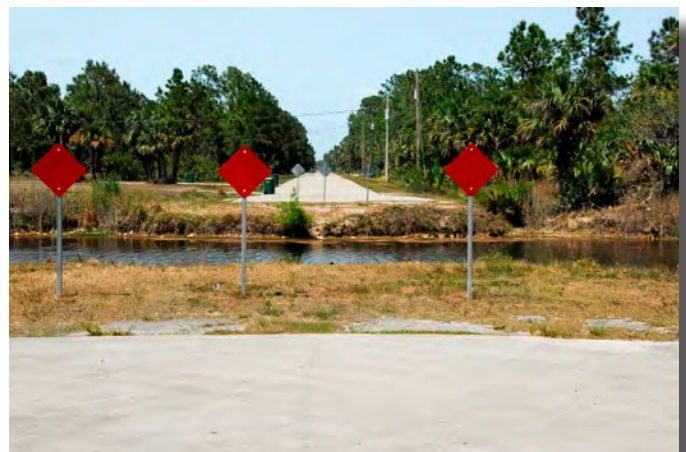
16th Street NE - truncated at canal (photo courtesy of Stantec)
