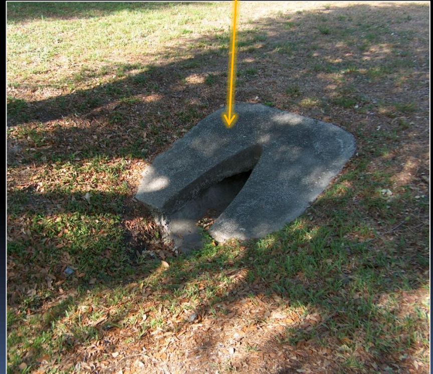
Concrete apron protecting pipe end
