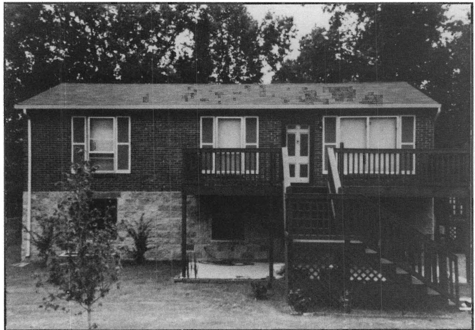
Figure 5: Example Of A Home Raised With The Brick Veneer In Place — Completion.
