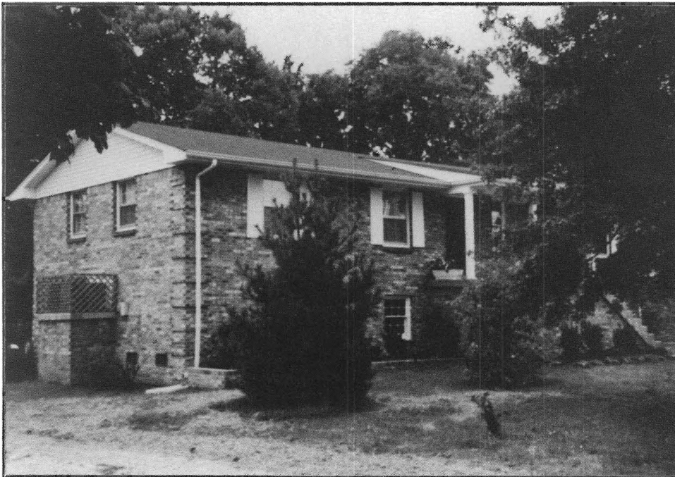
Figure 7: Example Of A Home Raised With Air Conditioner Compressor Unit On Elevated Platform.
