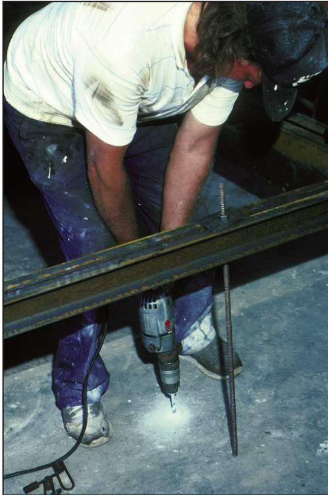
Figure 77 ... install anchors ...
