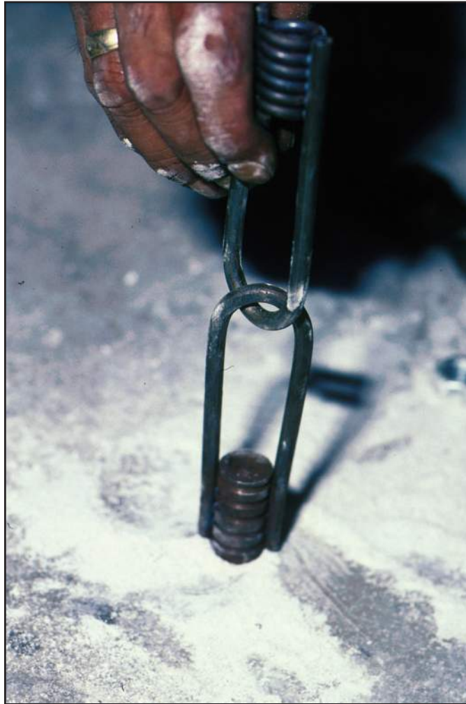
Figure 78 ... and use hangers to attach the anchors to the grid of steel beams.
