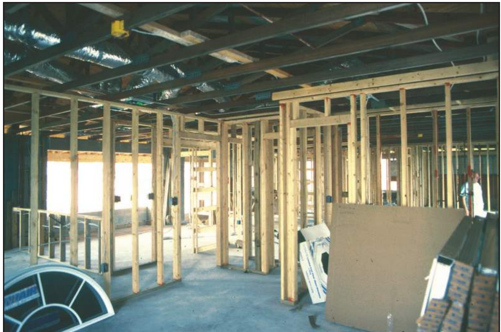
Figure 30 Interior partition walls and utilities are added.
