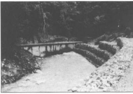
Structural techniques to modify channels and control stream flow include the construction of diversionary walls and gabions—prefabricated baskets of rock within wire cages used to stabilize banks.
