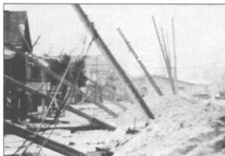
Hurricanes can cause severe damage due to the combined effects of several agents—high winds, increased wave action, heavy precipitation, storm surge, and other types of flooding.
