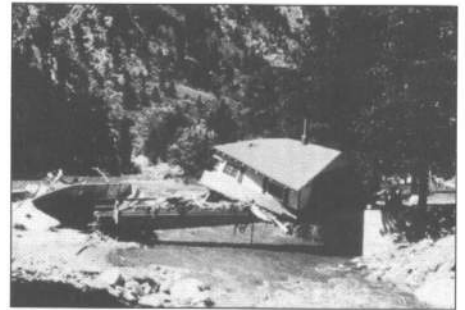
Big Thompson Canyon, Colorado, following flash flood, July 1976.
