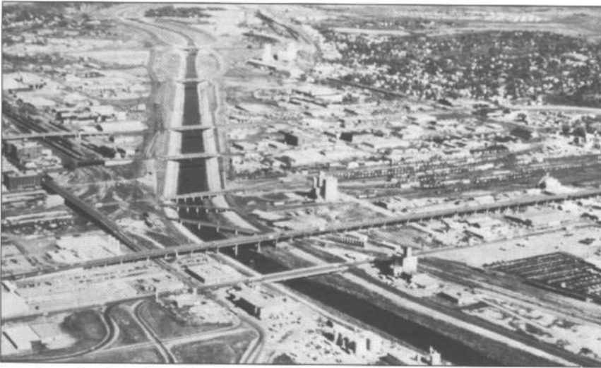
It has been estimated that 3.5 to 5.5 million acres of floodplain land had been developed for urban use by the late 1970s. In many cases, this change has resulted in greatly altered river corridors and adjacent lands. Channel modification, Sioux City, Iowa.
