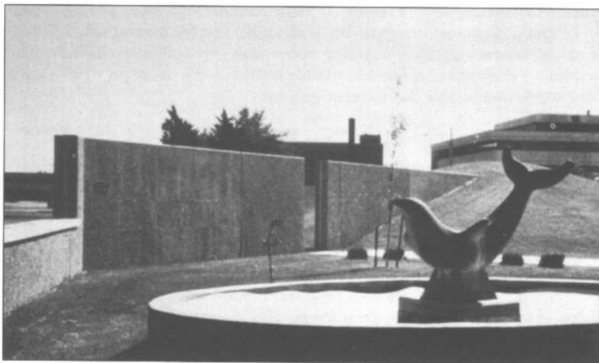
An estimated 25,000 miles of levees and floodwalls have been built nationwide. They can be very effective in reducing flood losses, although areas behind levees and floodwalls may risk greater than normal flood damage. Floodwall, Waterloo, Iowa.
