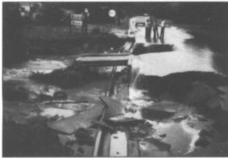
Damages to infrastructure may account for as much as 25% of the total damages incurred during flooding.
