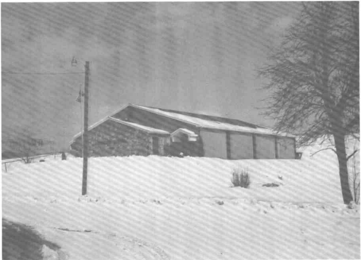
Structure elevated approximately 10 feet on earth fill for approximately 3% of the total project cost.
