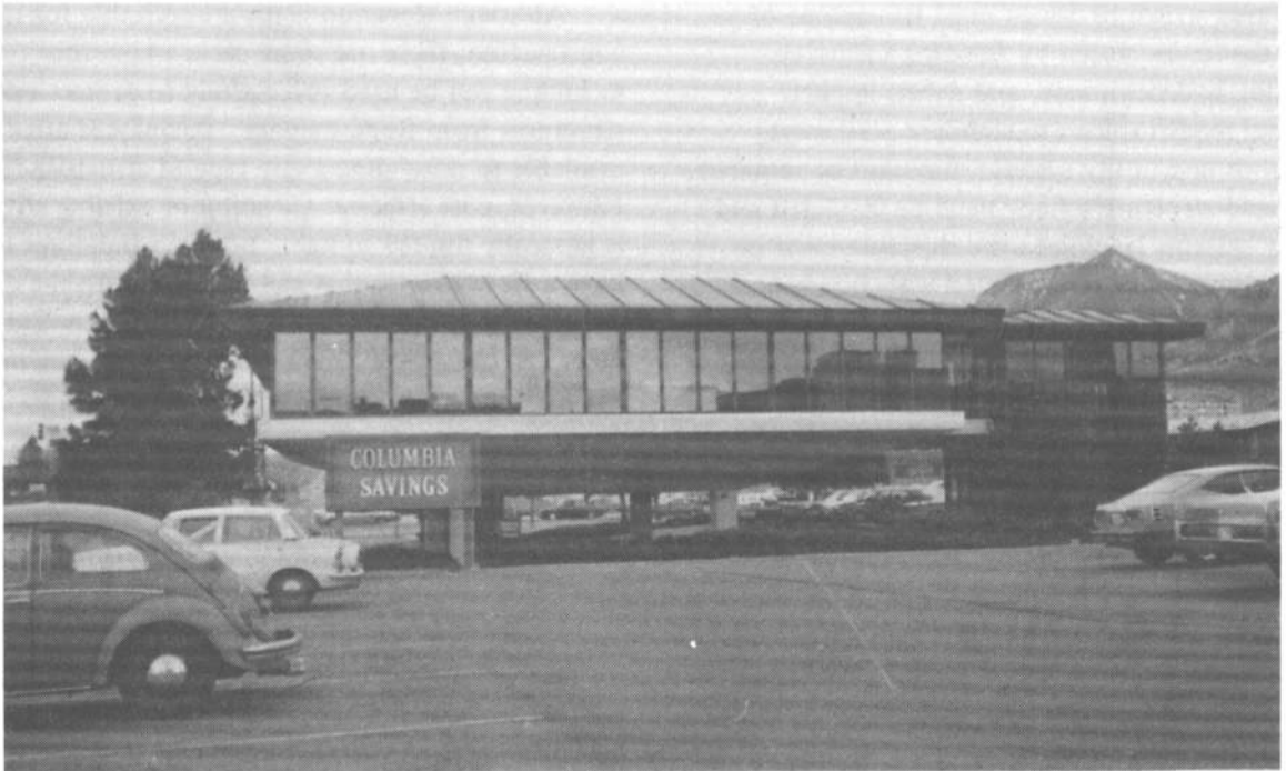
Figure I-7. Elevation on Columns
