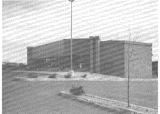
Site grading provides direct access to first floor elevation at the front of the structure.
