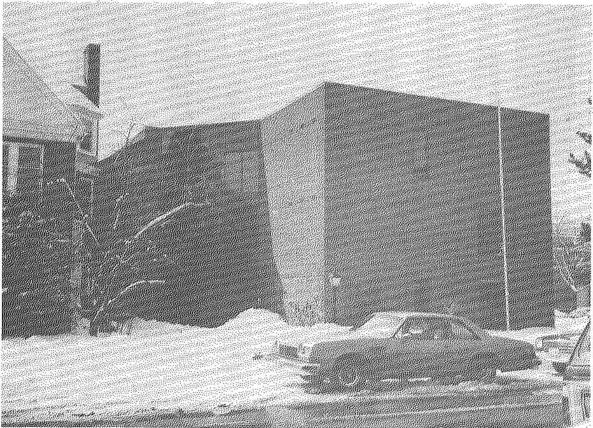
Structure has been elevated 7 feet above the base flood level in recognition of potential damage from floods that exceed the regulatory flood level.
