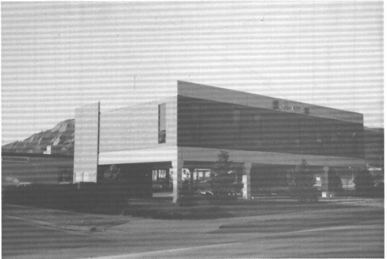
Figure III-4. Platform Construction Source: Elevated Residential Structures
