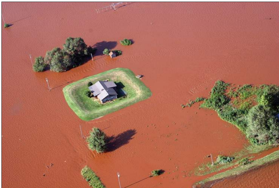
Figure 3-18. A home protected by a levee.
