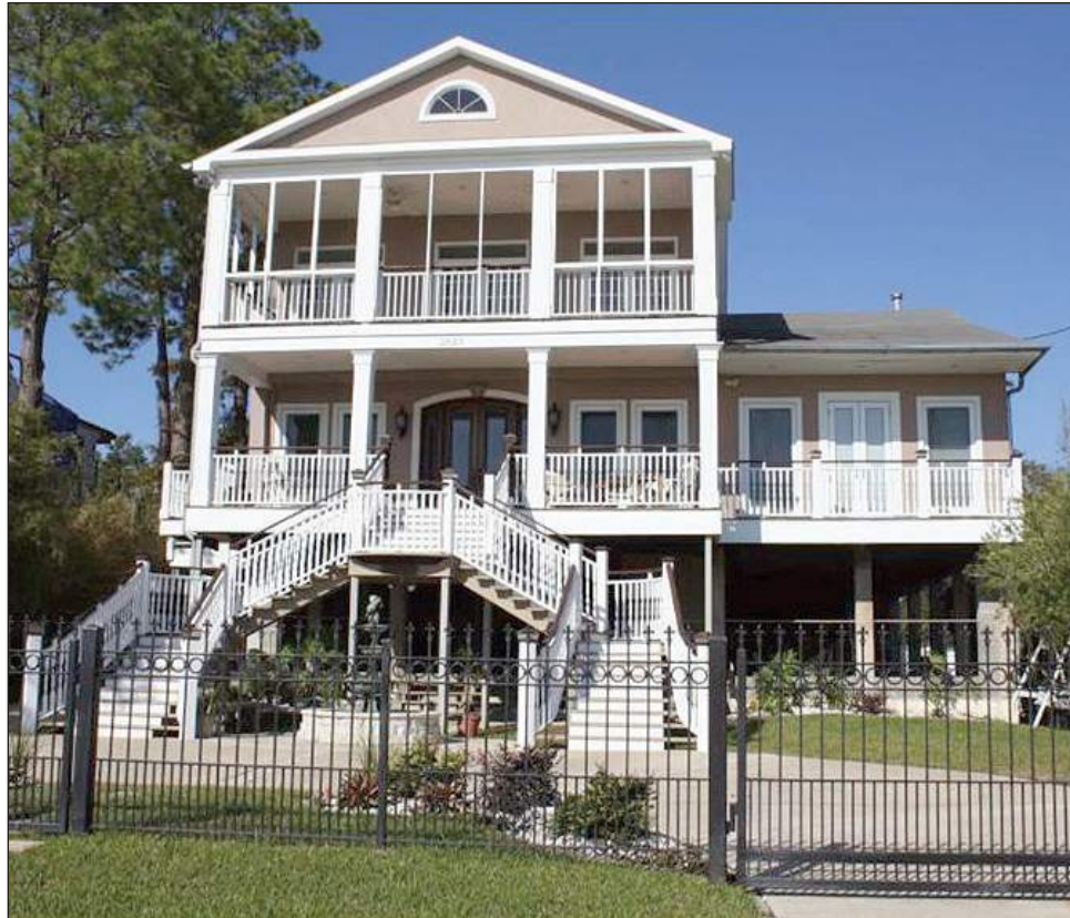
Figure 2-2. This home, from Figure 2-1, was elevated in a manner that added to both its appearance and its value. As a result of its elevation, the home avoided major damage from Hurricane Isaac in 2012.
