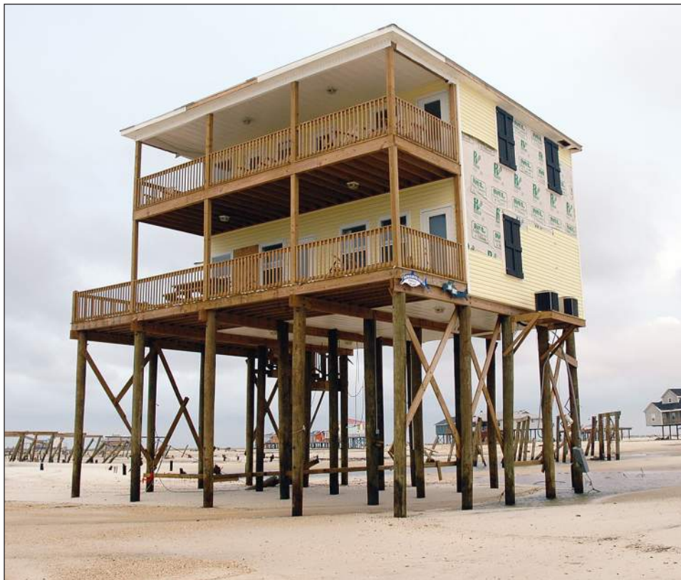
Figure 3-10. Home elevated on piles.
