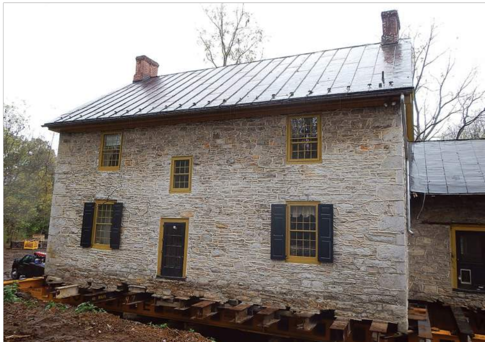
Figure 6-8. House is lowered and connected to the foundation after the foundation is fully constructed (photo courtesy of Wolfe House Movers).
