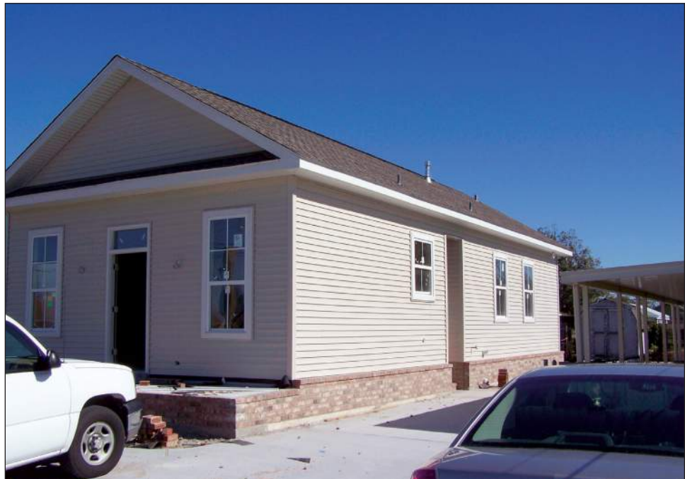
Figure 6-9. Typical mitigation reconstruction project.
