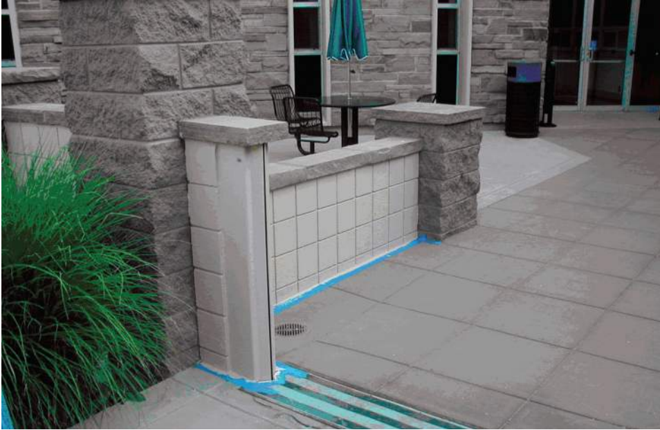
Figure 8-5. The City of Boulder, CO, installed a “pop up” closure to this floodwall at a City office building subject to flash floods. The closure floats up into place automatically when the site is flooded.
