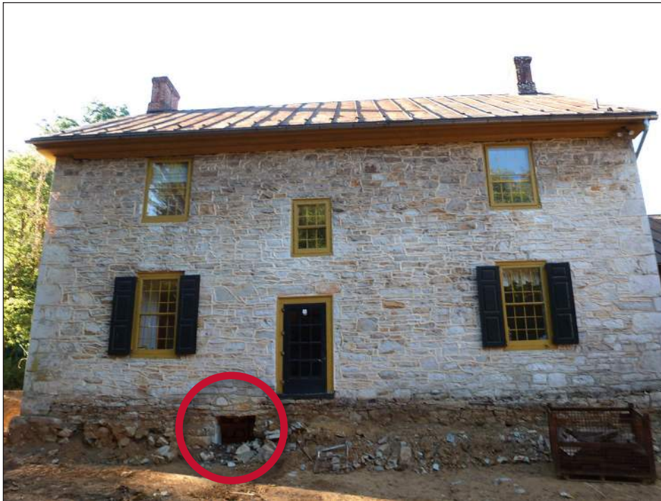
Figure 6-2. Clearing pathways beneath the structure for lifting supports (photo courtesy of Wolfe House Movers).
