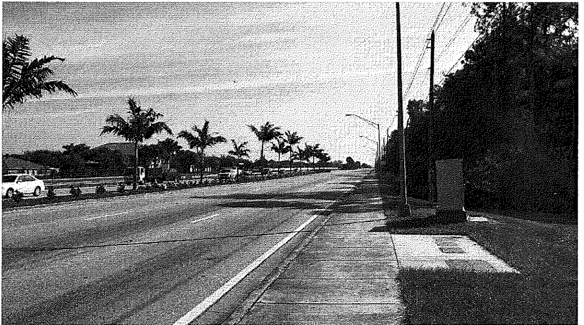
View east of Immokalee Road from Valewood Drive Extension. Subject to right of photo.
