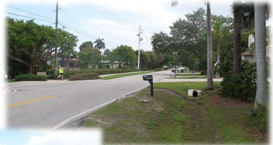
Photo 19- South Project Stormwater Enclosure.
