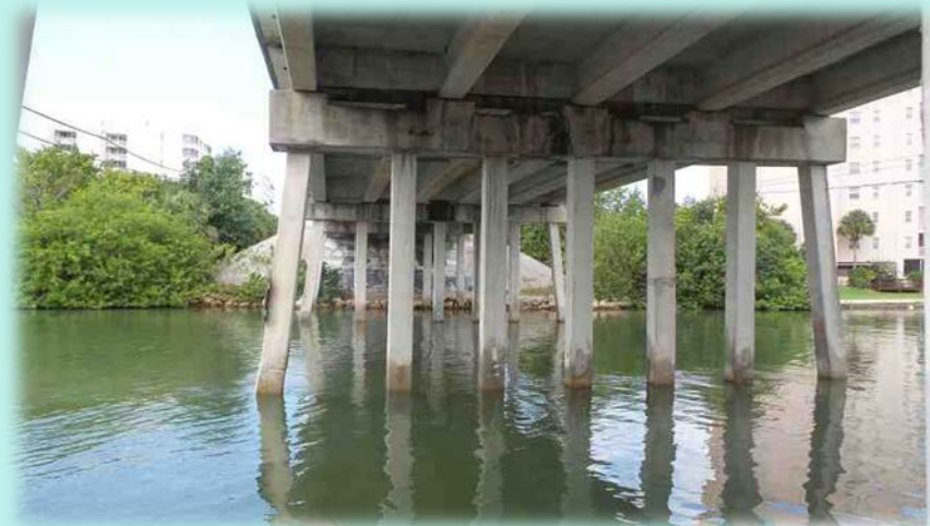
Photo 2 - Delnor Wiggins Bridge Piers
