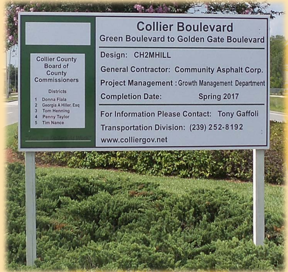
Photo 5 Collier III Phase I Under Construction
