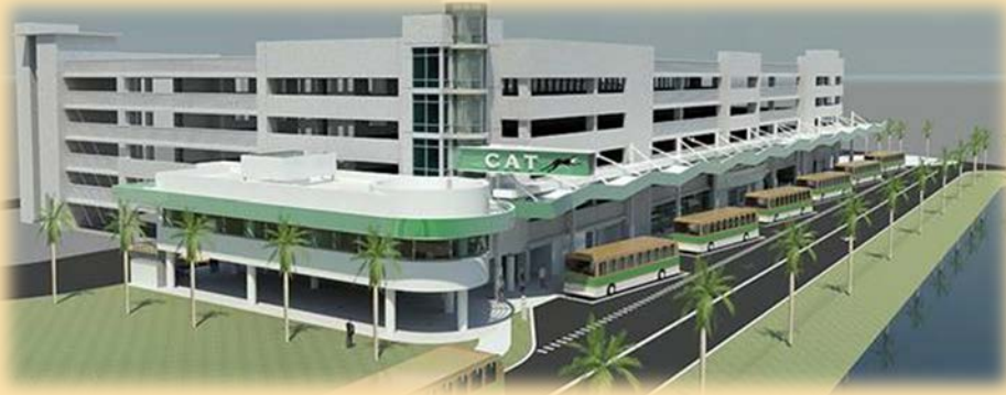
Photo 17 – Collier Area Transit Transfer Facility
