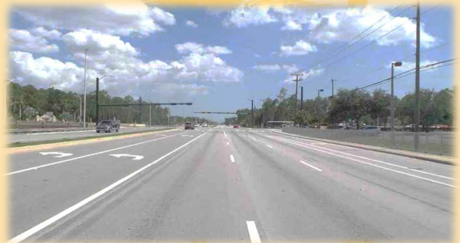
Photo 3-Completed Collier II Segment
