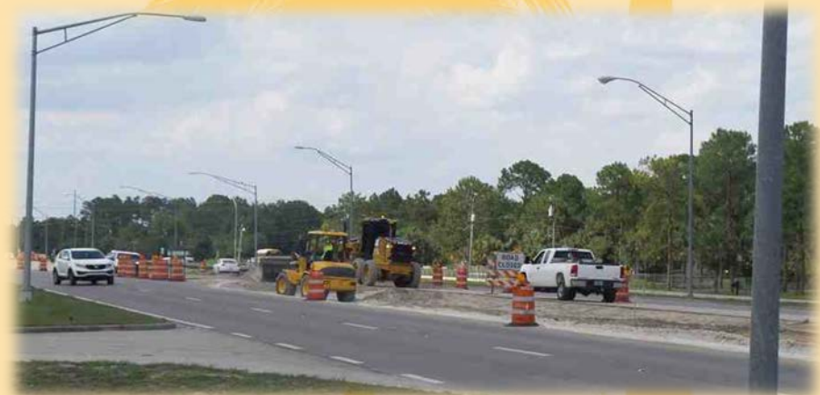
Photo 4- Construction on Collier III - Phase I
