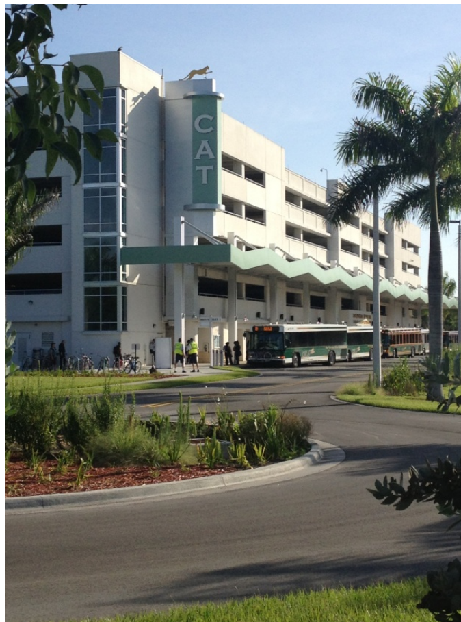
Figure 2-13 Intermodal Transfer Station
