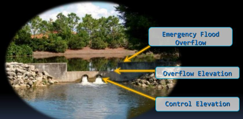
Structures should be checked regularly especially during the wet season, and cleared of debris. In some cases the structure openings may be under water making regular maintenance difficult but if the small "control" opening is obstructed water must rise higher to the overflow elevation before flowing out.
