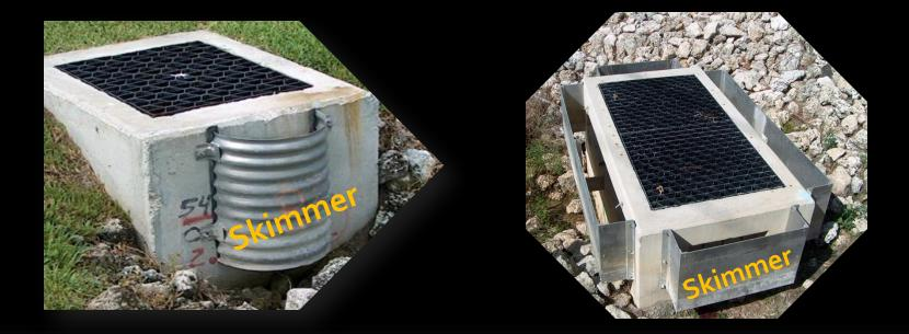
Skimmers keep floating debris from obstructing the flow of water out of a control structure, which might otherwise cause flooding.
