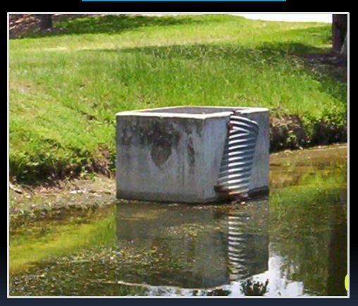
This skimmer is rusted at the bottom and falling off. It is not likely to be protecting the outlet hole so that water can exit the pond when the water level is high.
