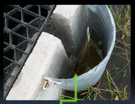
There should be a minimum of 1 foot of clearance under the skimmer so water fills from the bottom and can exit the **outlet hole**
