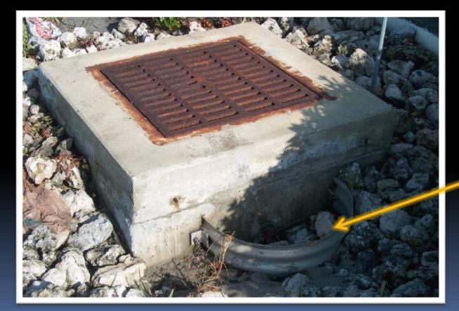
This skimmer does not have clearance at the bottom for the rising waters to exit, it is buried. There should not be sediment and rocks in skimmers.
