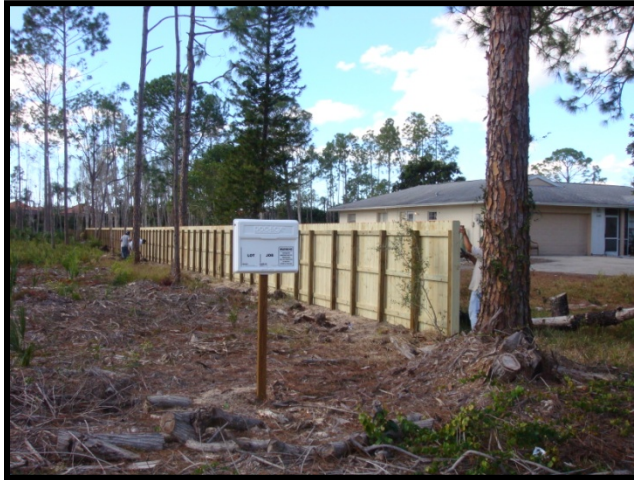
Six-foot high, wood privacy fence along the eastern half of the northern boundary of the Logan Woods Preserve. Photo by Christal Segura
