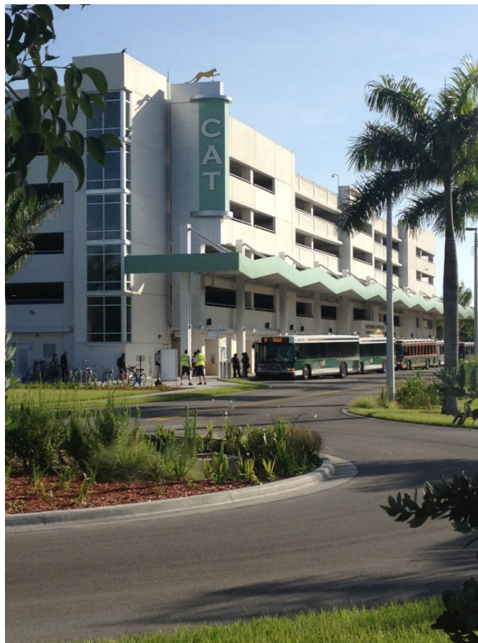
Figure 2-13 Intermodal Transfer Station
