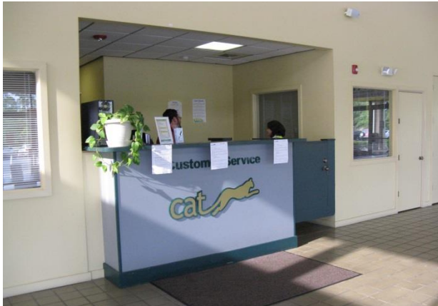
Incompliant desk height
