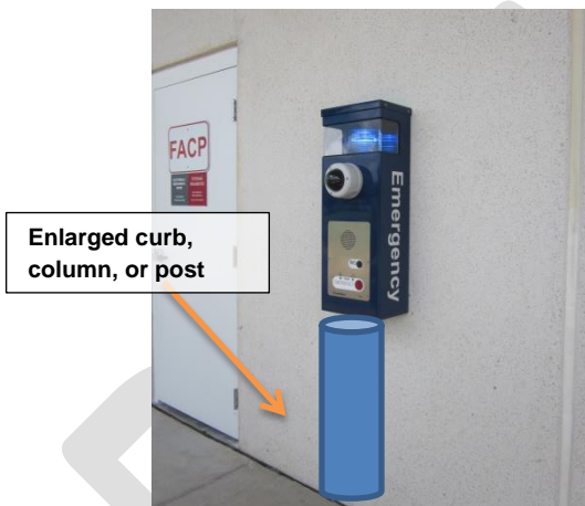
This emergency assistance box is a protruding object
