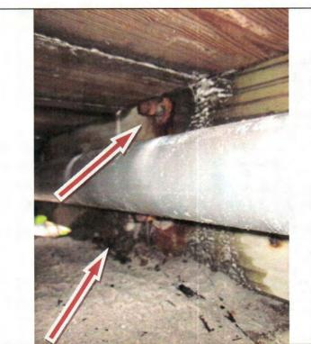
**ISSUE:** Electrical conduits and small water pipes are strapped to the stringers with plastic straps or in some cases plastic hangers. Note the corroding washers and complete loss of hex-nuts, of both of the thru-bolt connectors, to corrosion, at the base of a rail post over Pier #3. The anchor bolt and clip angle appear to have completely corroded away as well.
