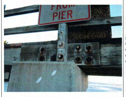
**Description:** View of an identical splice assembly at Pier #6, past the stair landing opening, where extra pairs of thru-bolt are used to stiffen up the outside stringer past the stair landing opening on the left.
