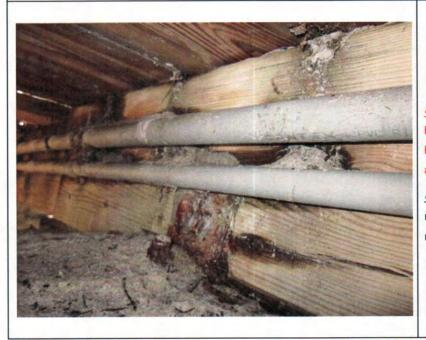
**Issue:** View of an inside stringer anchor bolt/clip angle assembly which is normally buried under the beach sand causing accelerated corrosion of the metal hardware. **Resolution:** Regular inspection and replacement of deteriorated hardware is required.
