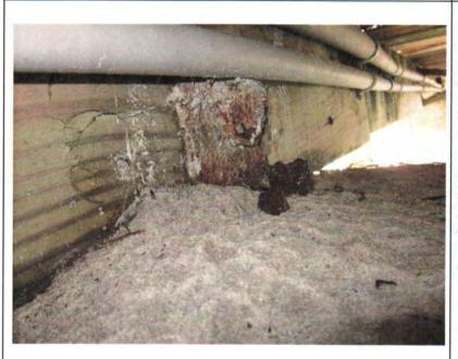
**Issue:** View of an inside stringer anchor bolt/clip angle assembly which is normally buried under the wet beach sand and debris causing accelerated corrosion of the metal hardware.
