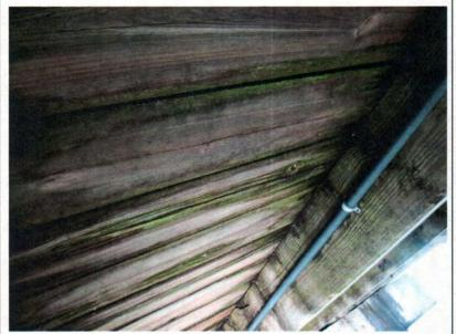
**Issue:** In stormy day and high waves the deck is being washed in sea spray for the duration. Note the boards are soggy from such weather event. Note board with split fiber in the center.
