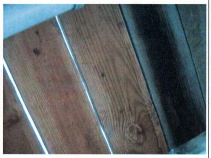
**Description:** Typical view of the substructure framing and the condition of the decking in the vicinity of Pier #12. Note the multiple replacement boards besides the old boards.
