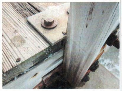
**Issue:** The connection assembly on the pier is the most vulnerable to sea spray that brings split and decay on wood, and promotes accelerated corrosion of metal hardware.
