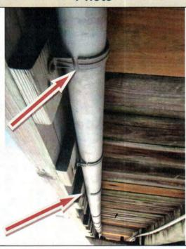
**Issue:** The stress caused by the movement of the main power supply conduit is beyond the working strength of these thin plastic pipe straps.
