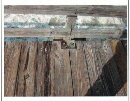
**Description:** View over Pier #20. As the pier begins to go over water seaward, the impact of the sea environment is increasingly harsh on wood and metal hardware. Note the sign of decay on the board immediately to the left of the post. Note a decaying board on the left.
