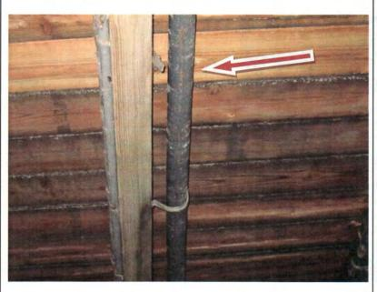
**Issue:** Pier #11-Pier #12. The stress caused by the movement of the main power supply conduit is beyond the working strength of these thin plastic pipe straps.
