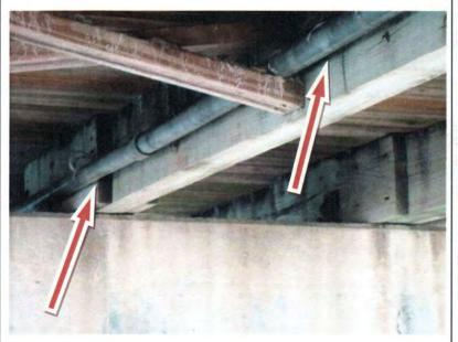
**Issue:** The stress caused by the movement of the main power supply conduit is beyond the working strength of these thin plastic pipe straps.
