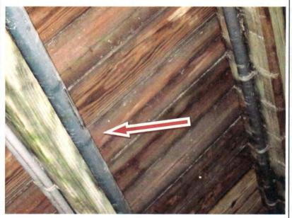
**Issue:** Pier #11 – Pier #12. The stress caused by the movement of the main power supply conduit is beyond the working strength of these thin plastic pipe straps.
