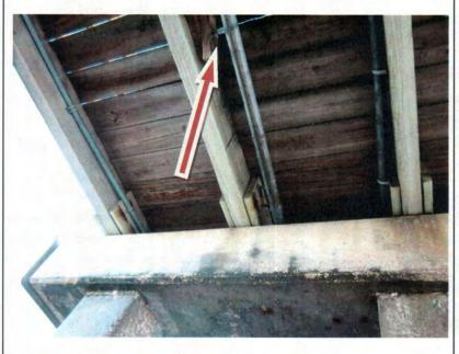
**Issue:** The stress caused by the movement of the main power supply conduit is beyond the working strength of these thin plastic pipe straps.
