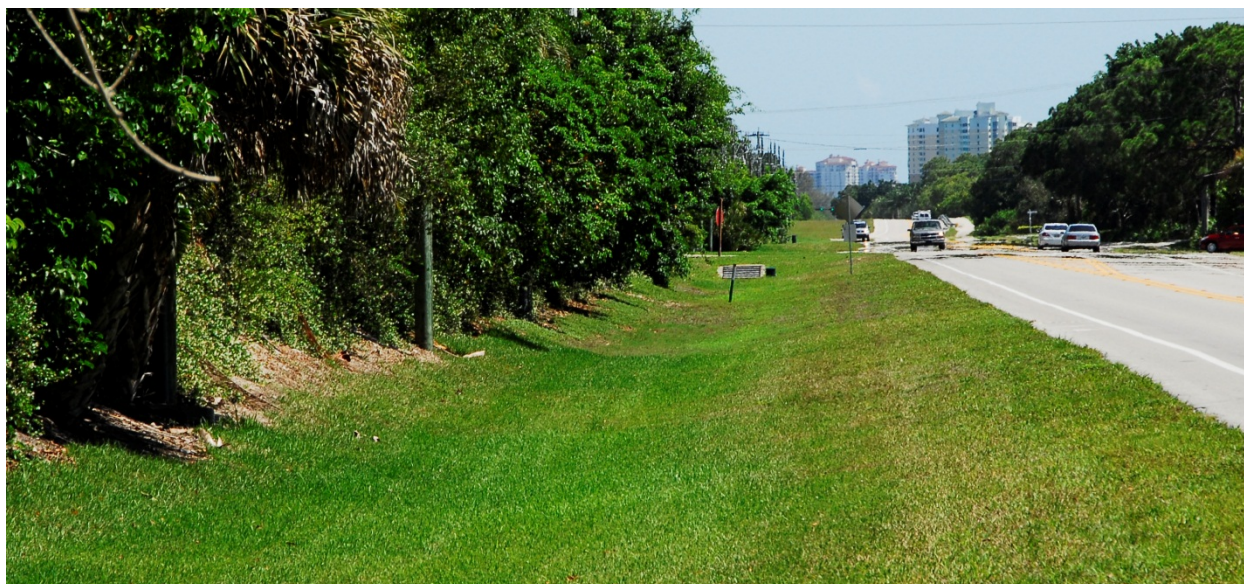
FIGURE 22: Roadway Drainage Swale
