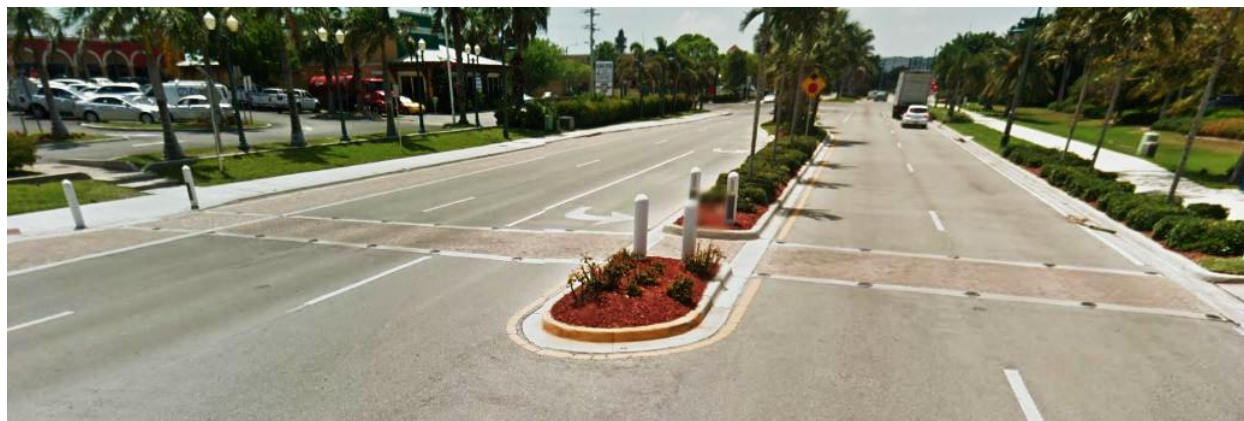
FIGURE 15: Example Mid-Block Pedestrian Refuge Island
