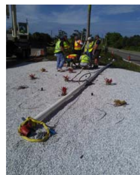
Pump & drop pipe pulled
